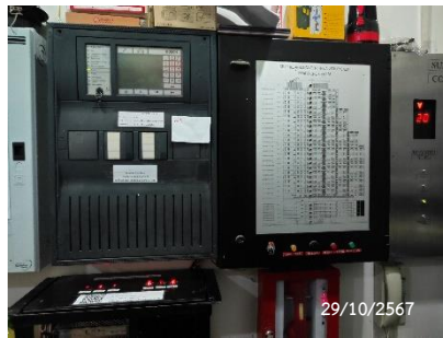
Fire Alarm Control Panel
